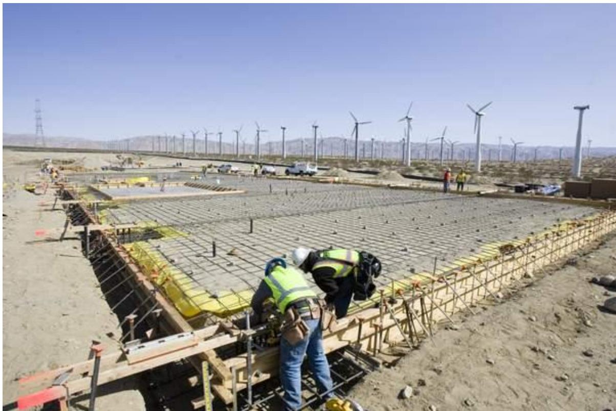
Workers build a foundation at the CPV Sentinel peaker power plant. The plant, which would be able to run up to 116 days a year, will have eight General Electric LMS-100 turbines that each will be able to produce 100 megawatts. / Omar Ornelas, The Desert Sun
